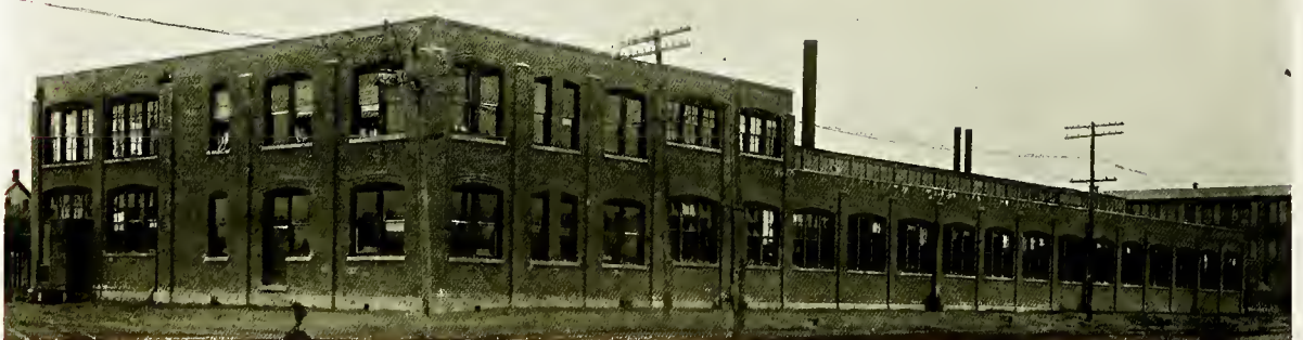
The Adler Machine Co. Plant (Located at Kingston). A Suburban Industrial Concern
